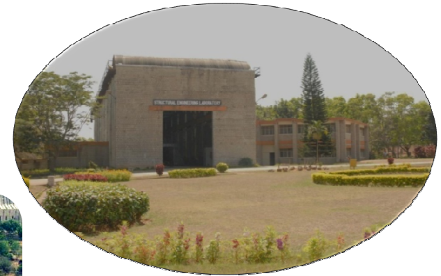
STRUCTURAL ENGINEERING LABORATORY
